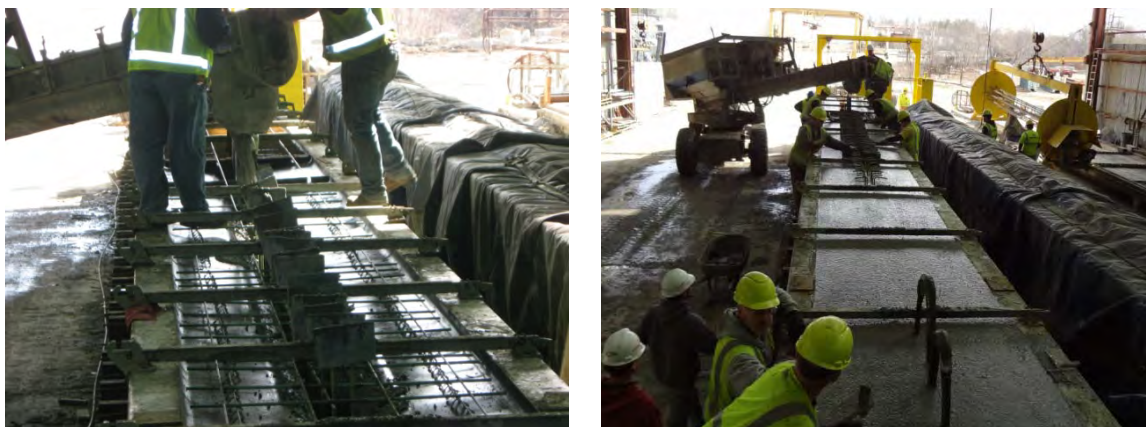
Figure 5-11. Fabrication of Test Girders
