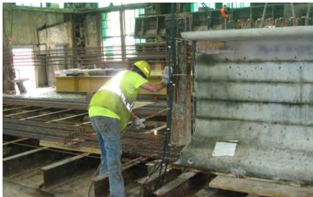
Figure 5-55. Release of PC/PS Girder
