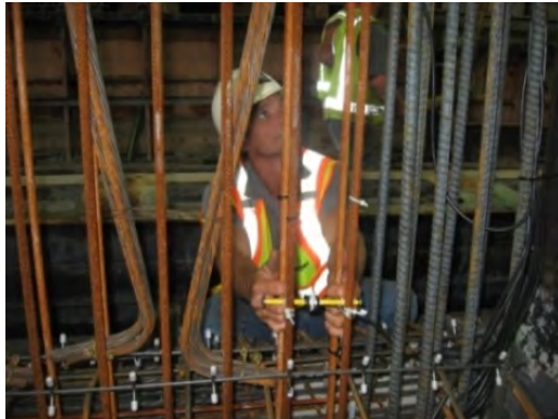
a) VWSG Installation at Specified Depth
