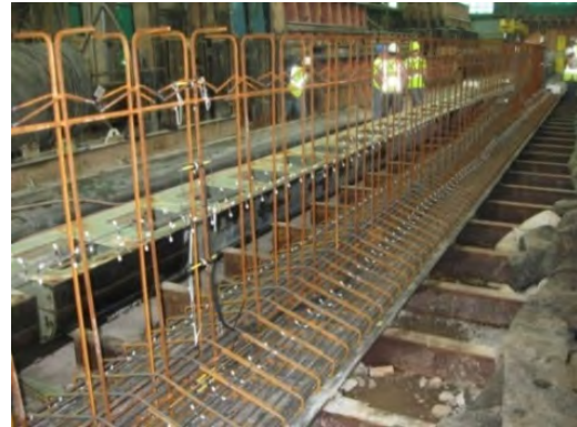
b) VWSG Installed at Specified Sections
