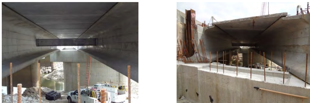
Figure 5-62. Diaphragm and PC/PS Panels Erection
