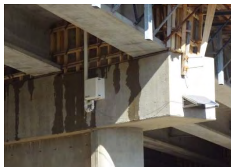
d) CR800 DAS Anchored to Bent 3 Pier Cap
