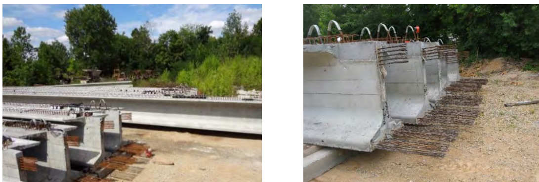
Figure 5-56. Girders Storage at Precast Plant
