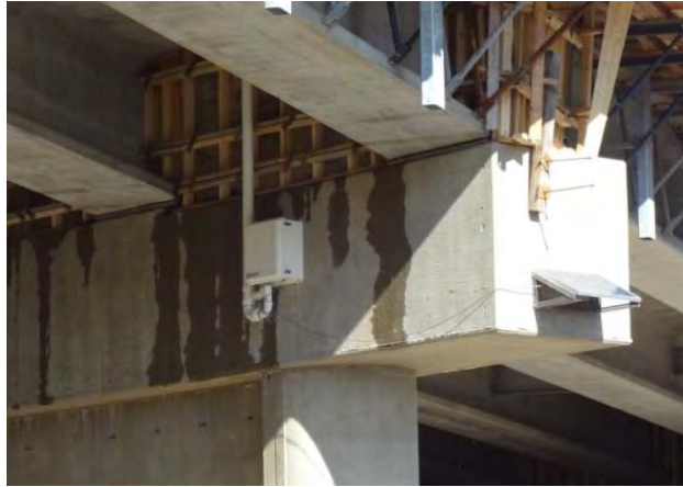
Figure 5-43. Bridge A7957 VWSG Instrumentation
