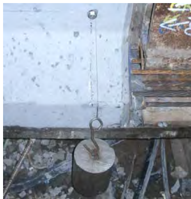
Figure 4: Dead Weight for Tension-Wire System
