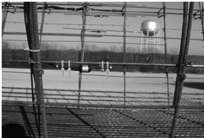
Figure 1: Instrumented Vibrating Wire Strain Gauge (VWSG) on Prestressing Strand
