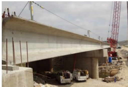
Figure 5-60. Conventional Concrete and HS-SCC PC Girders Placed on Supports
