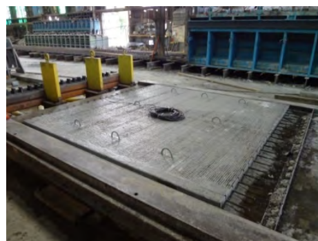
b) After Concrete Placement
