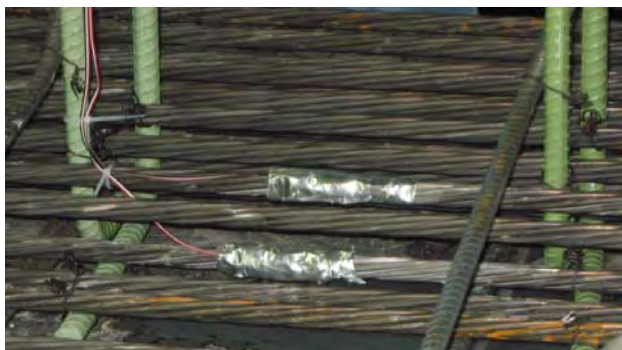
Figure 5-10. Strain Gauge Installation
