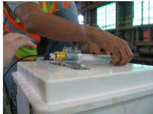
b) Antenna Installation to DAS Box 1
