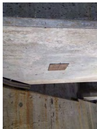
b) Steel Plate Fixed (Girder's Bottom Flange)
