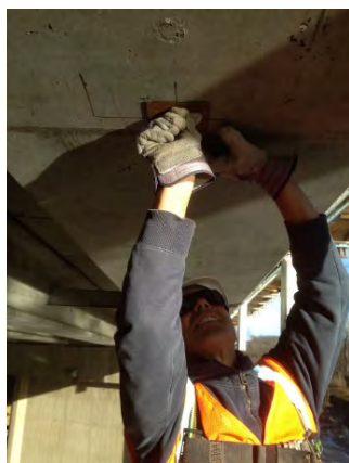
a) Steel Plate Installation
