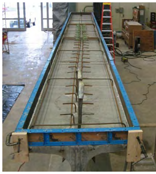
Figure 5-18. CIP Deck Preparation
