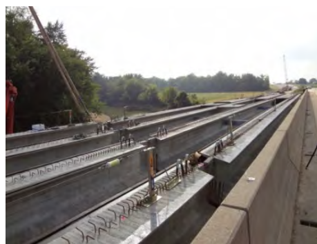
b) PC/PS Girders Placed on Their Supports
