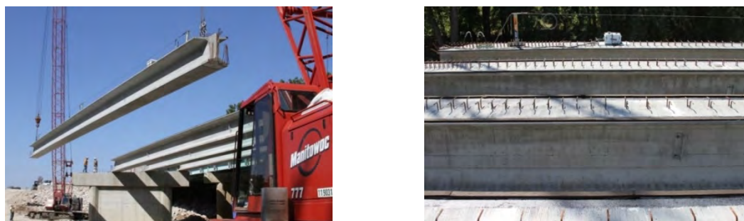
Figure 5-59. Lifting of HS-SCC PC Girder 4 (Span 2-3)
