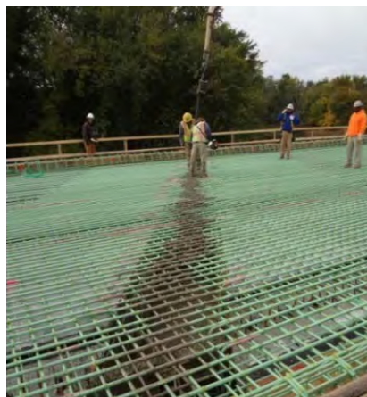
Figure 5-64. Concrete Placement on Intermediate RC Diaphragm
