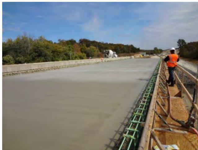
Figure 5-67. Finished Surface of CIP RC Deck
