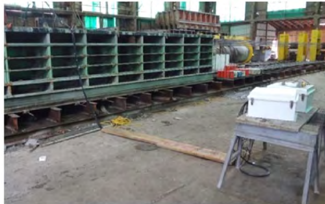
Figure 5-54. Data Collection During the PC/PS Girders Fabrication
