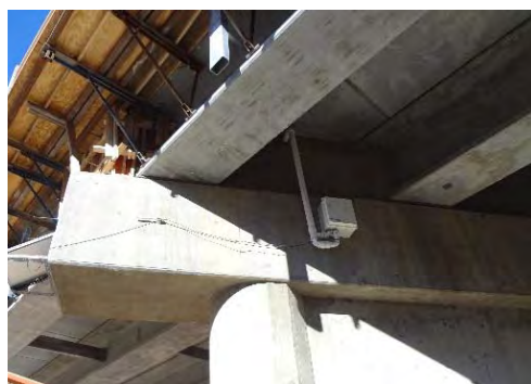
a) CR800 DAS Box Installed on Bent 3
