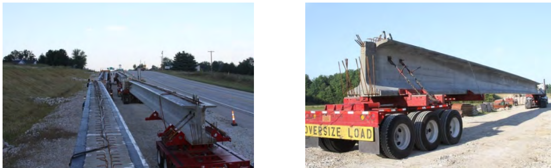
Figure 5-57. Shipping of the PC Girders to the Bridge Jobsite
