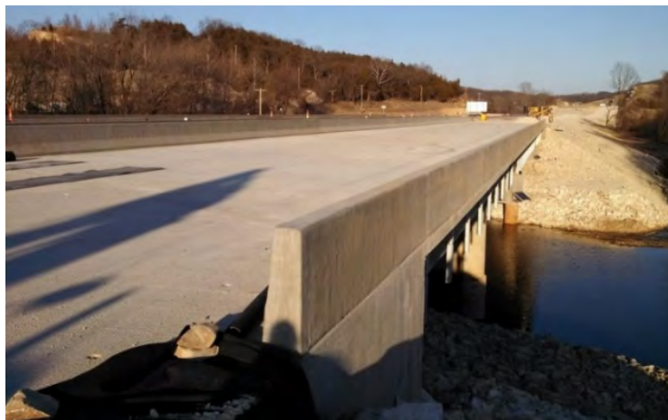
Figure 5-70. Bridge A7957 Completed
