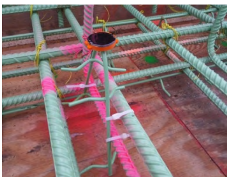
Figure 5-47. RFID Installed on CIP RC Deck (Before Concrete Placement)
