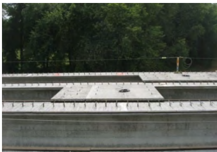
Figure 5-41. Instrumented PC/PS Panels
