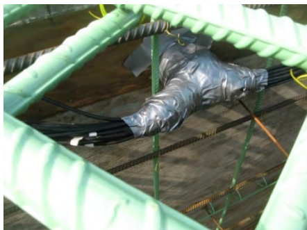
a) VWSG Wires Passed through Formwork
