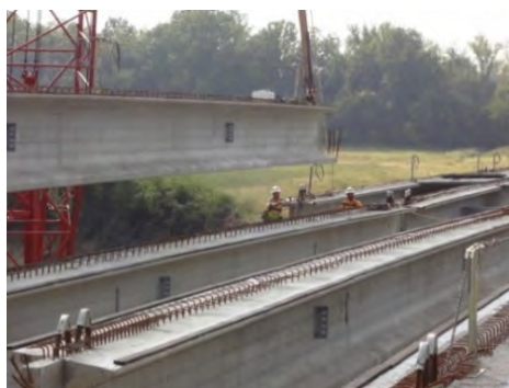
a) NS-SCC PC/PS Girder 4 with DAS
