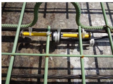
a) Before Concrete Placement
