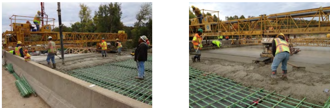
Figure 5-65. Concrete Placement on CIP RC Deck
