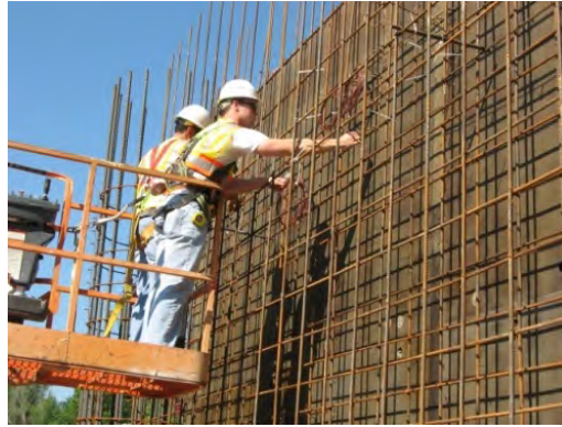
Figure 5-35. Thermocouples Installation on Bent 2's Web Wall
