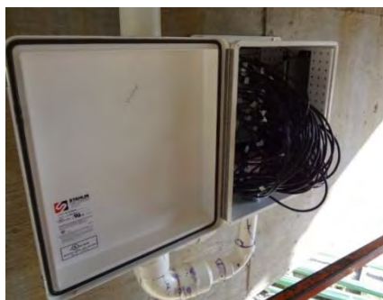
c) VWSG Wires Connected to CR800 DAS Modules
