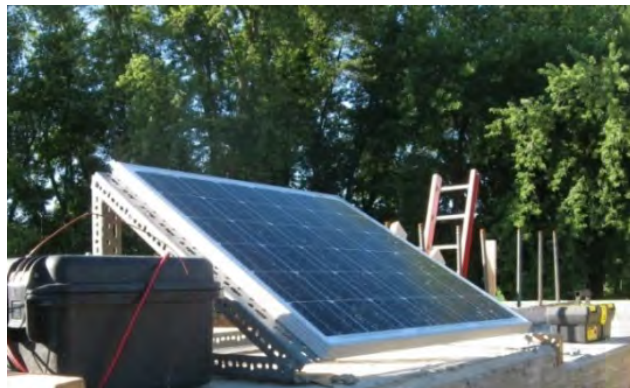
Figure 4-11. Compact RIO System and 90 Watt Solar Panel
